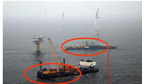
Infield cables on drums
