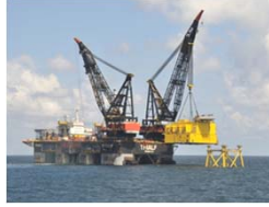
Installation of Offshore HVDC Converter Station
